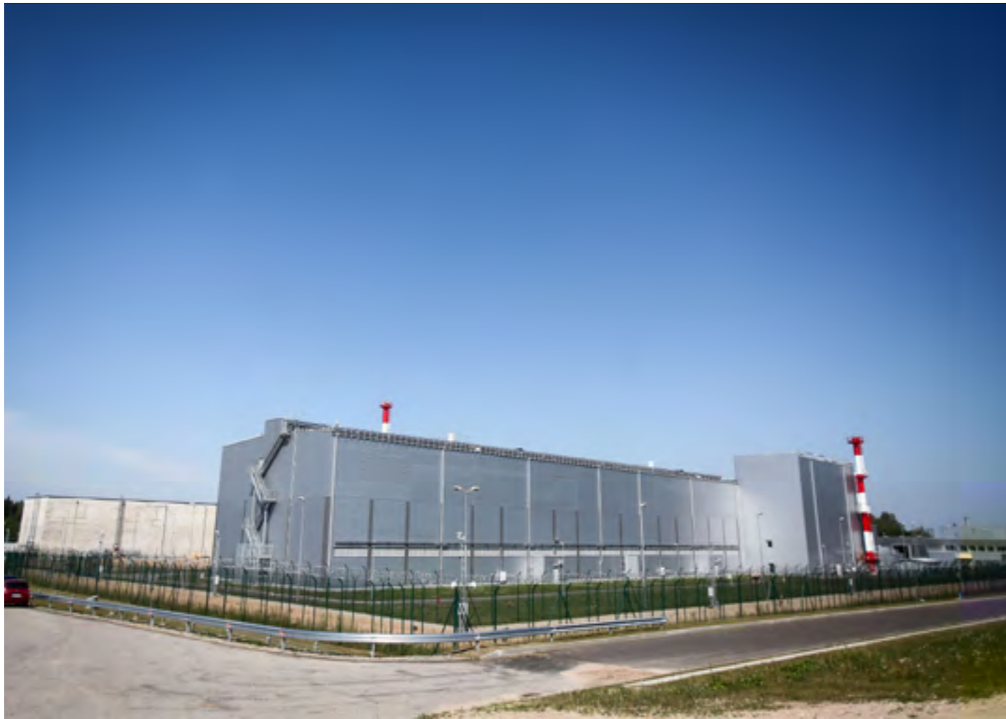
Laikinoji panaudoto branduolinio kuro saugykla New spent nuclear fuel storage facility
