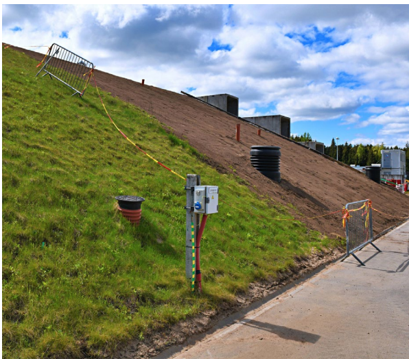
Mound of the very low level radioactive waste repository
