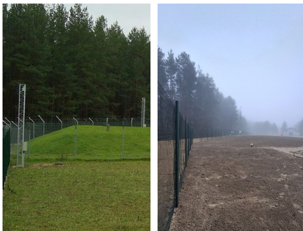
Maišiagala Radioactive Waste Storage Facility in 2021 and 2026
