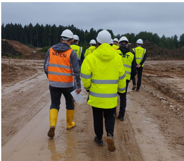
Inspection of the repository for low- and intermediate-level radioactive waste under construction
